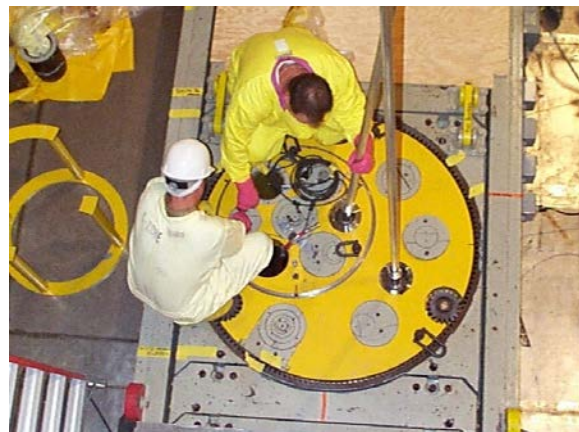
Fig. 8. Maintenance shield with rotating plugs used at ORNL.
